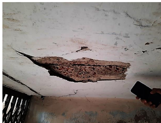
Fig. 3.11 Condition of the URM building's slab beneath.
