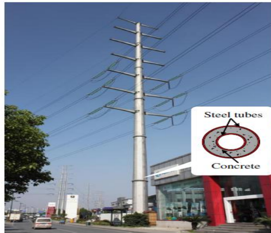
(c) A CFDSST electrical pole
