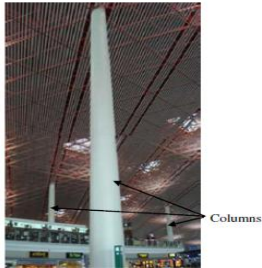
Fig 2.11 A practical application of CFT column with high slenderness ratio (An et al., 2012)
