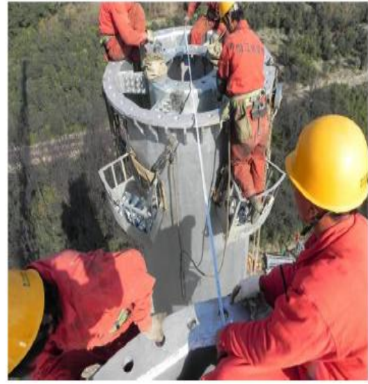
(b) Wind turbine installation
