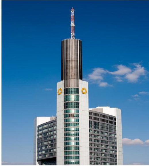
(a) Commerzbank Tower, Frankfurt
