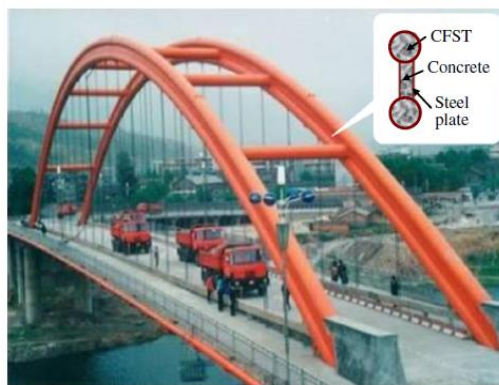
(c) Wangcang East River Bridge
