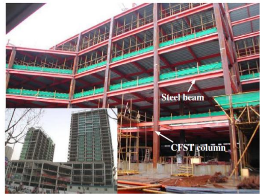
(b) Ruifeng building in Hangzhou
