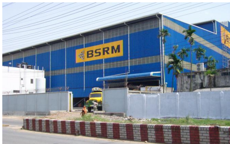
Figure 2.1 : Steel Melting & Billet Casting Plant, BSRM
